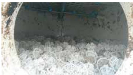
Replacement of Raschig Ring
