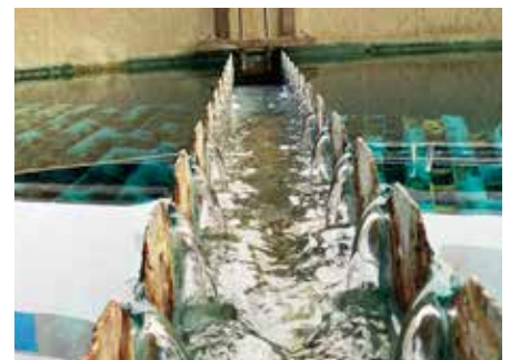
Water outflow from the sedimentation tank
