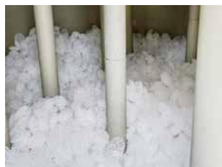
Backfilling scrubber towers with cleaned filters
