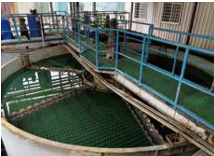
Sedimentation tank
